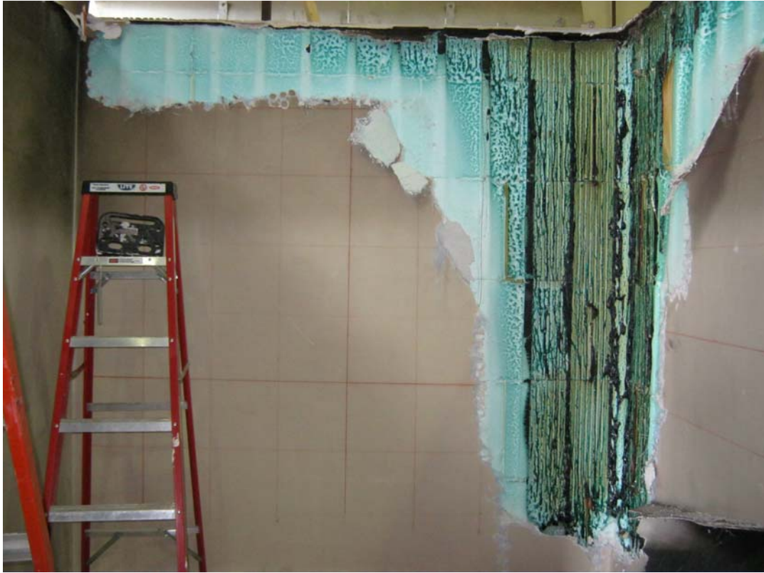
Post Test Photo with Plaster Removed
