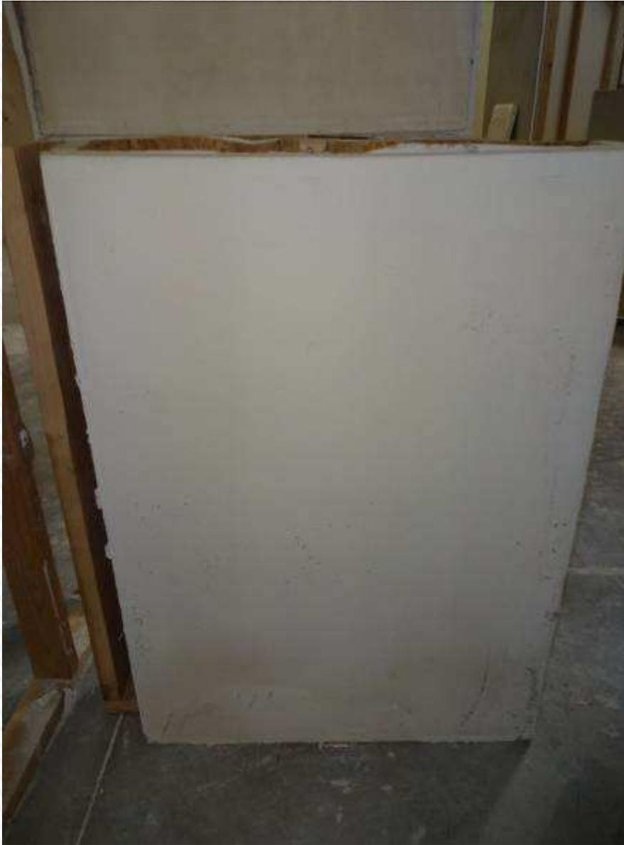
**Backside of the same wall, not even a crack or bulge in BallistiCrete.**
